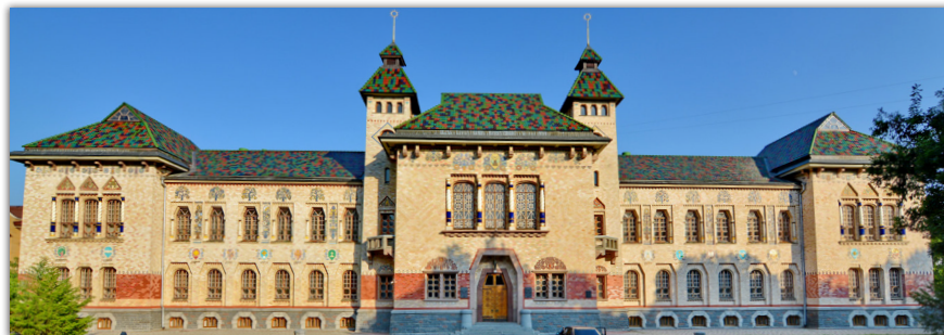
Fig. 17. The building of Vasyl Krichevsky Poltava Museum of Local Lore (former Natural Science Museum of the Poltava Zemstvo)
